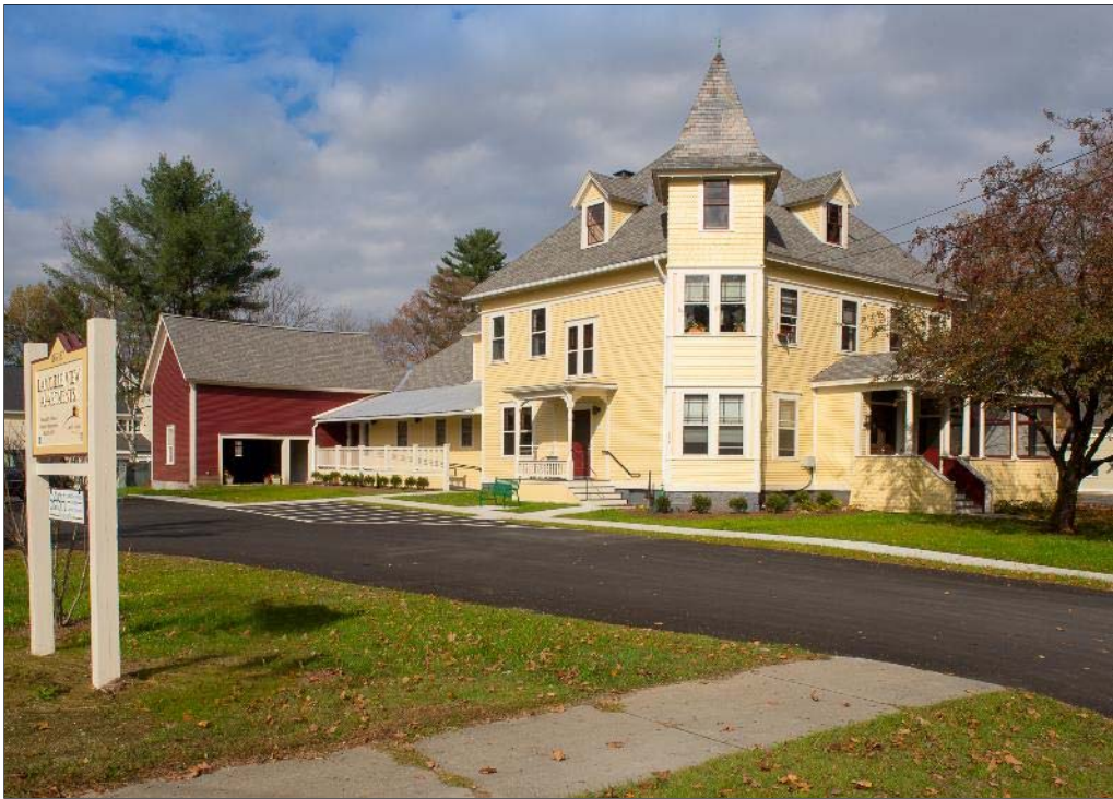
Lamoille View Housing, Morrisville
